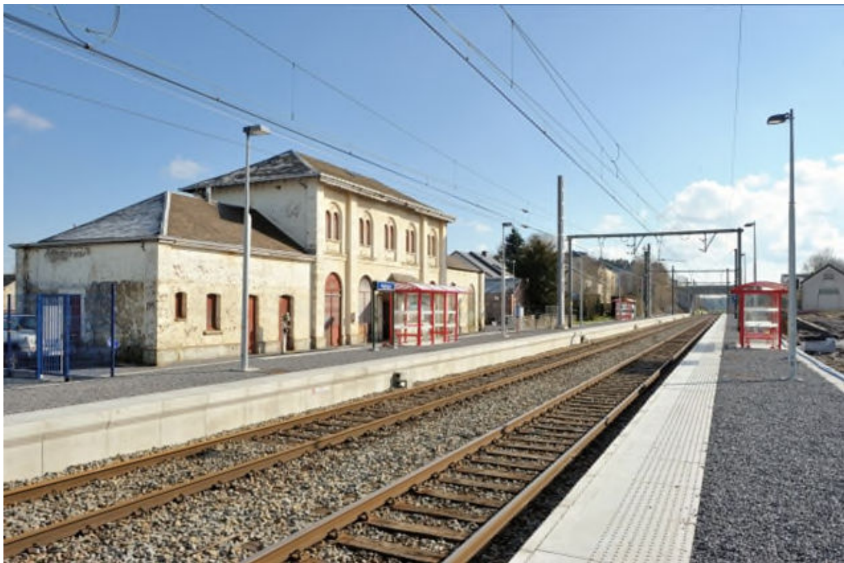
Station Habay, Denis Moinil, 2016. (Ref. D4142-6)
